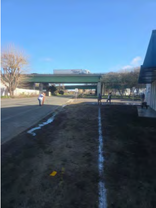
Office – beginning of the landscaping
