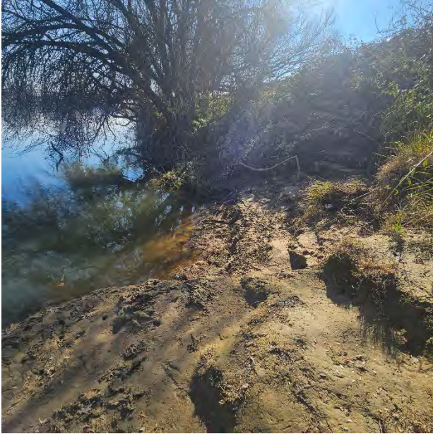
Erosion along the Sacramento River (currently under water)
